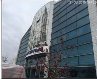
External photo(s) of the production unit(s) Outside view of the building.JPG
